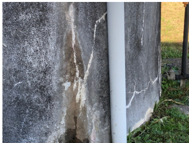
Cracked water tank that no longer holds water, on Italia Road, Balickera
